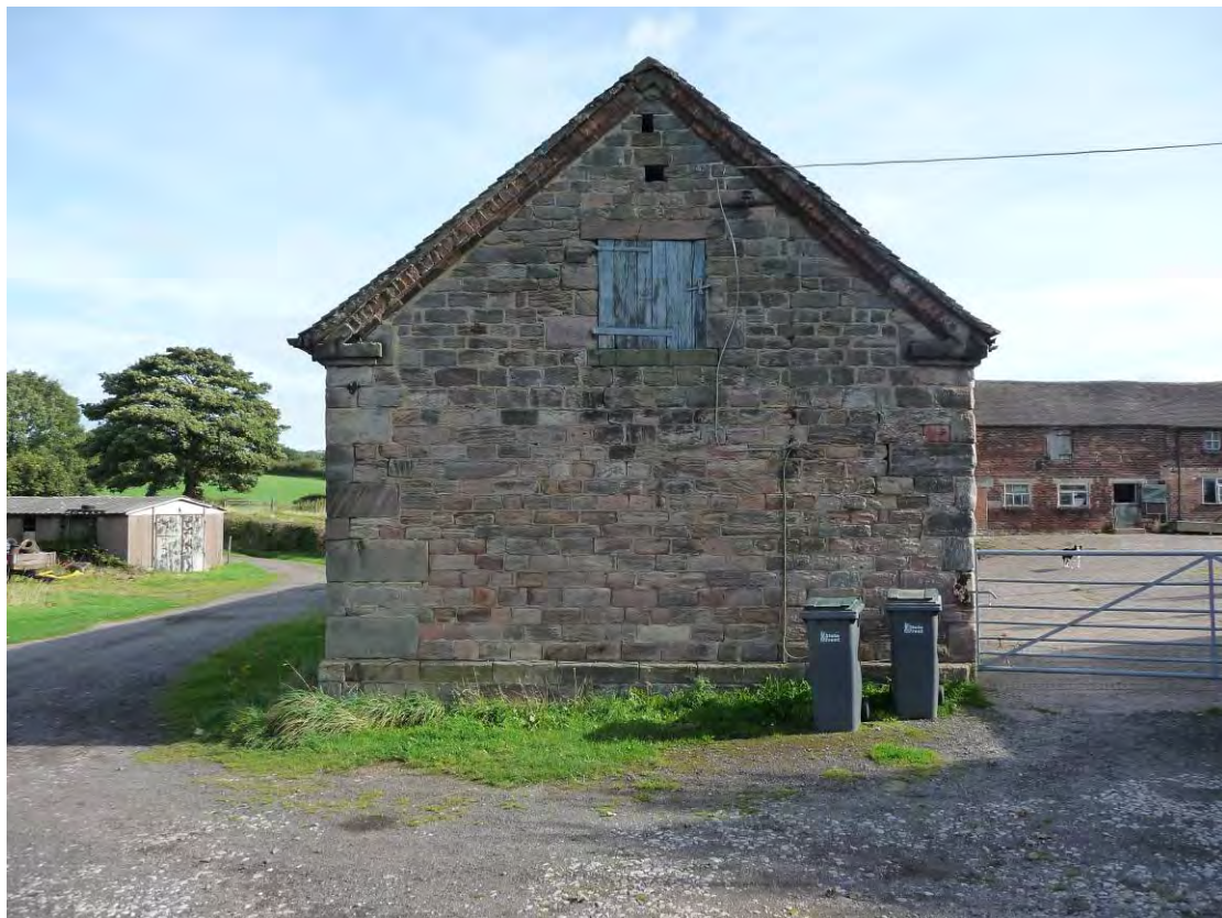
Fig. 38: Stone gable to farm outbuildings
