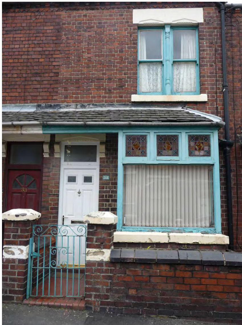
Fig. 8: Elevational detailing on No. 35 Harcourt Street
