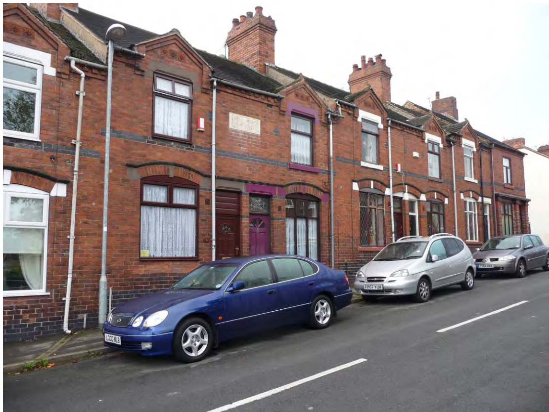
Fig. 34: View of front elevations to Foxley Terrace, Hardman Street
