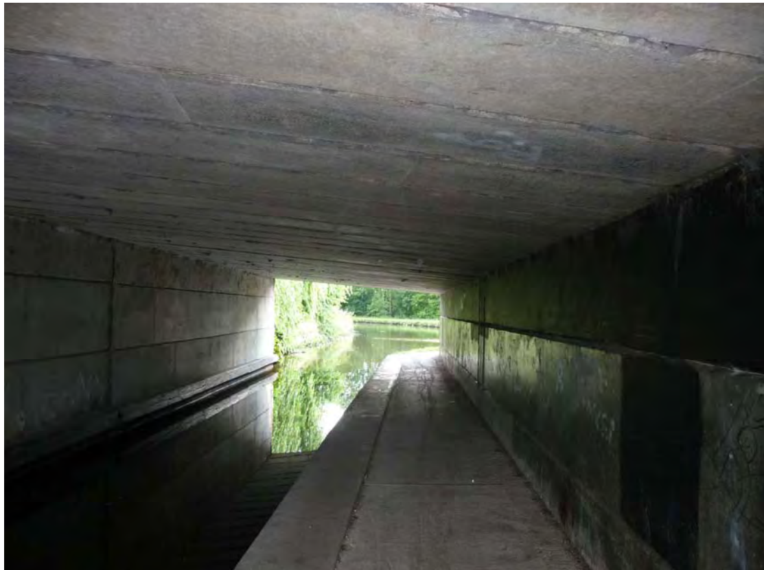
Fig. 25: The canal towpath passes under bridge 12
