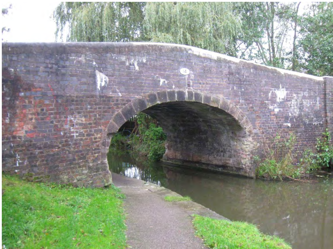
Fig. 28: Bridge 14 demonstrates traditional engineering techniques
