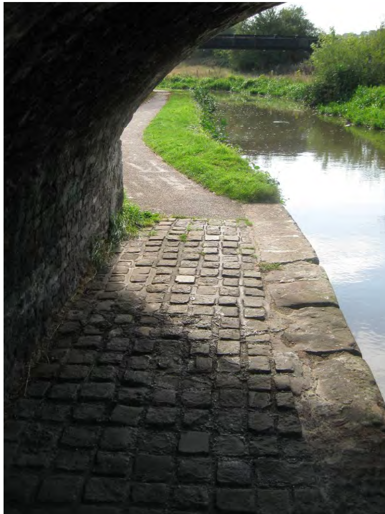
Fig. 30: Stone sett paving and edging to the underside of bridge 15
