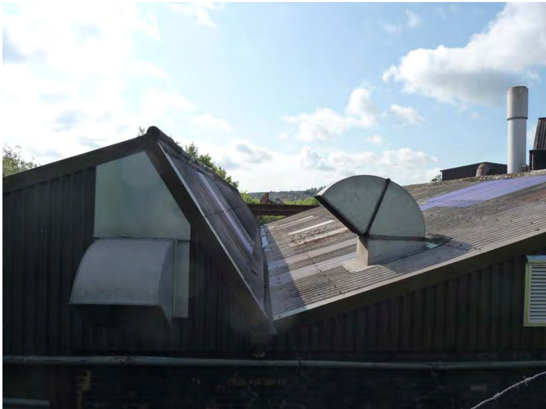
Fig. 22: Roofscape of canal-side industrial premises
