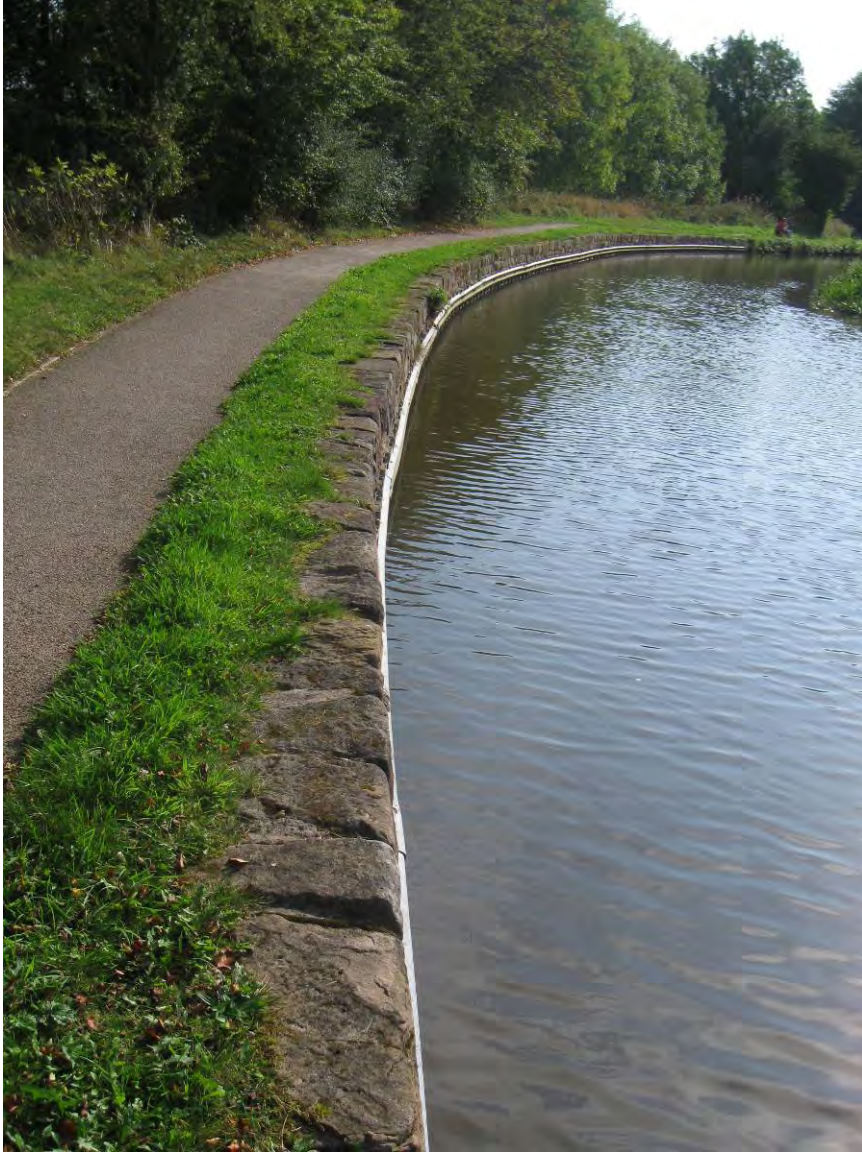
Fig. 31: Stone edging to canal towpath
