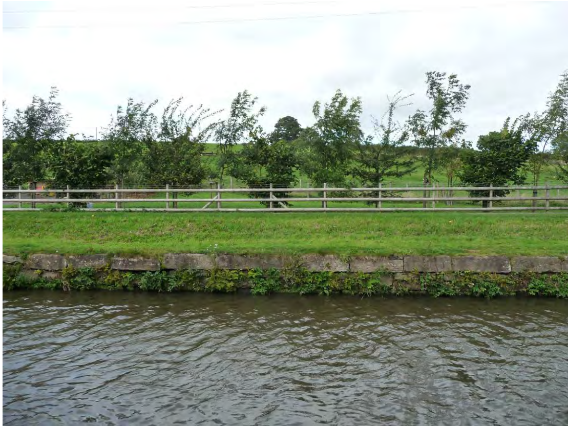
Fig.41: Original stone edging to canal edge
