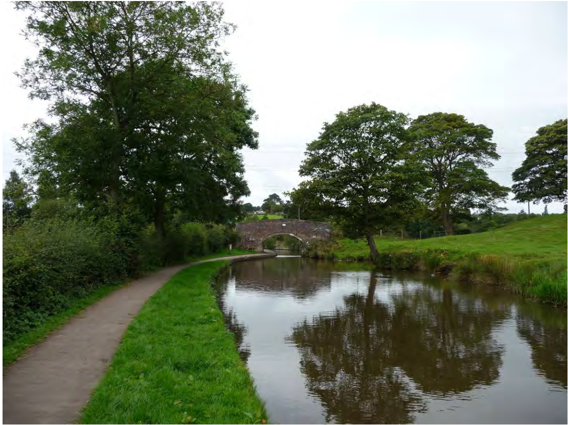
Fig. 43: Rural landscape setting to bridge 22
