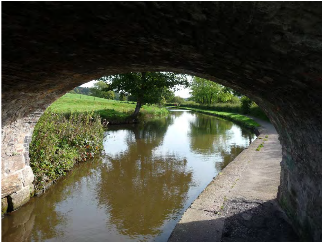
Fig. 37: View from bridge 22, looking east
