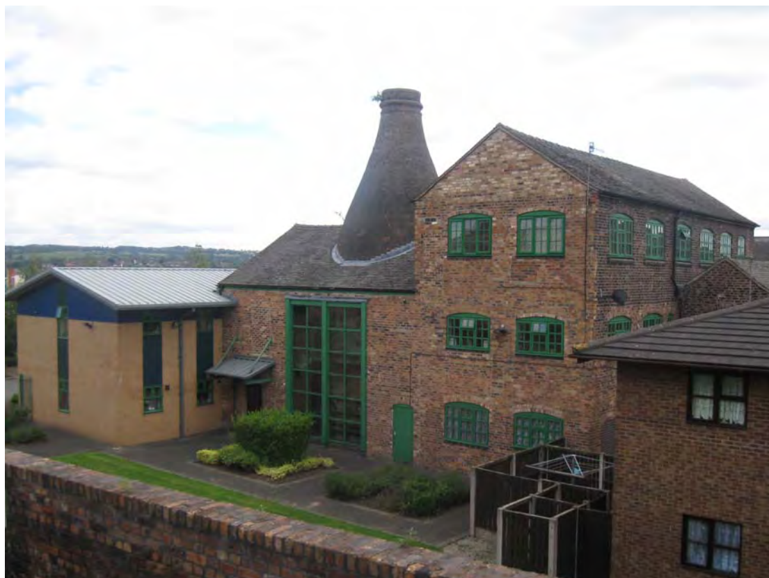
Fig. 19: Bottle oven contained within the fabric of the former potbank off Lichfield Street
