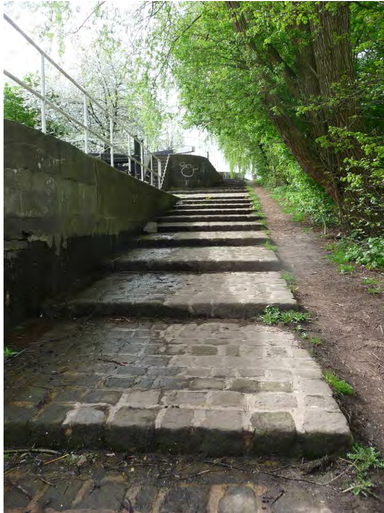
Fig.6: Stone steps to side of Bedford Locks
