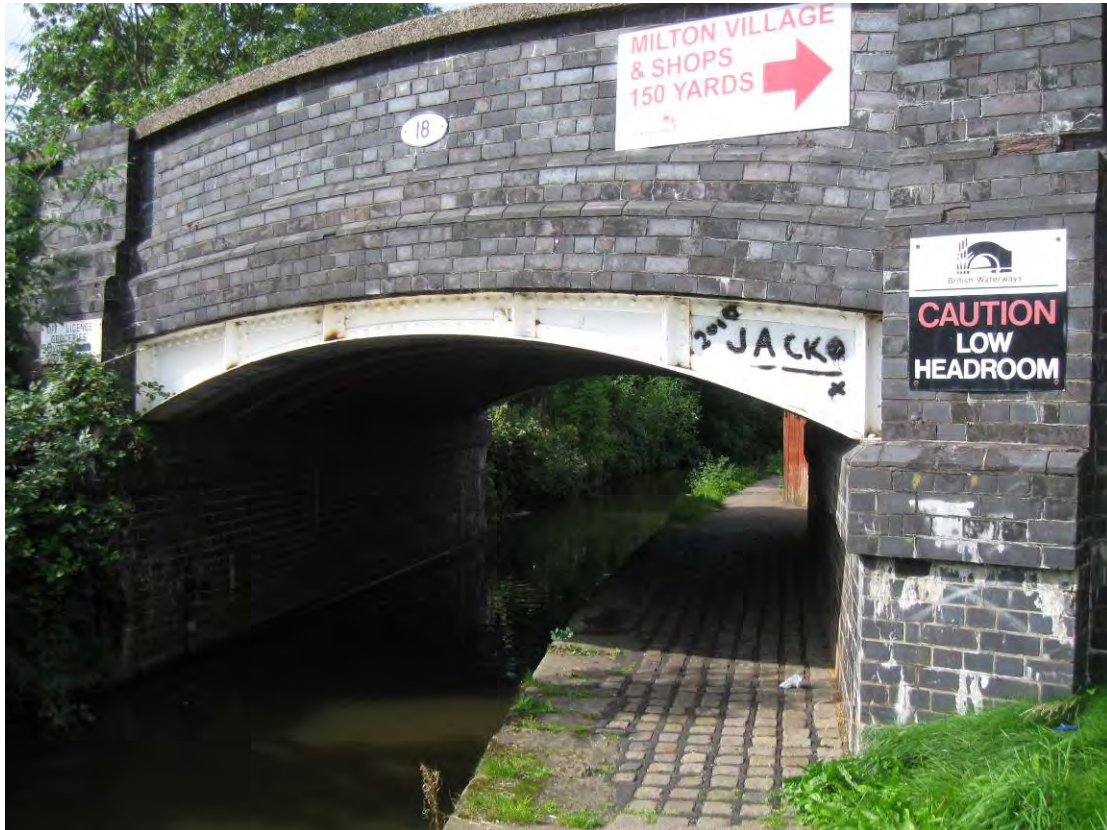
Fig. 32: Bridge 18, Milton, with stone setts to towpath
