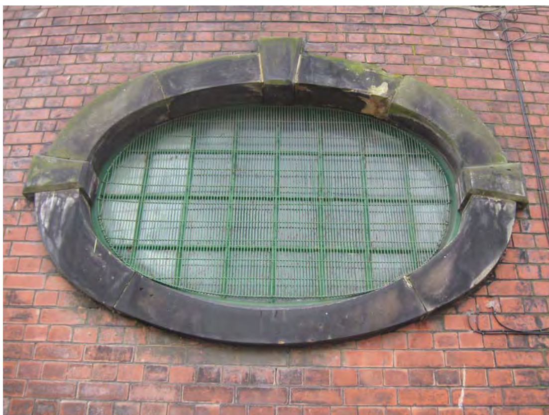
Fig. 15: Oval shaped window with stone surround and metal crittal windows
