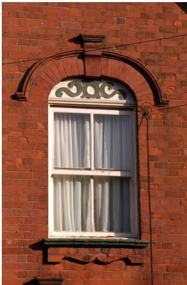
Figure 16: Windows with moulded aprons curved arches and prominent key-stones.
