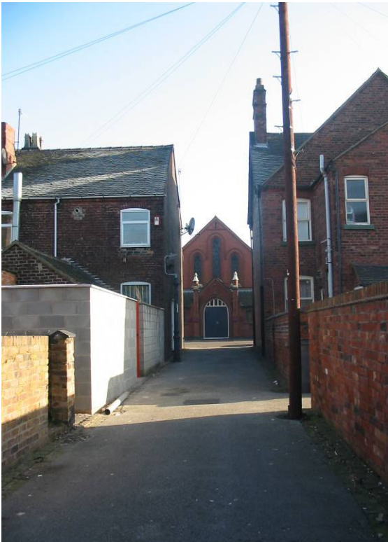
Figure 9: Alley way to side of conservation area.
