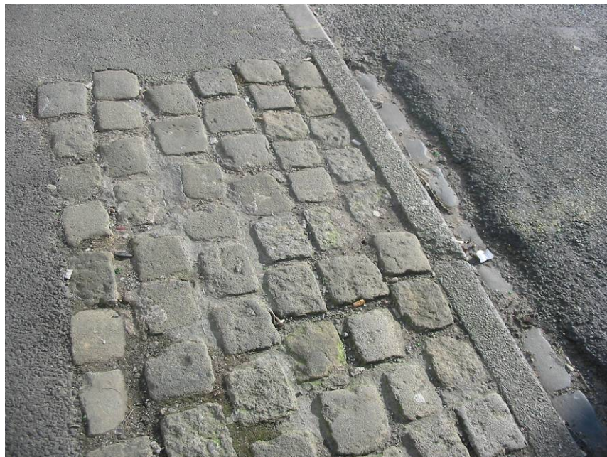
FIGURE 20: Fragment of original cobbled surface
