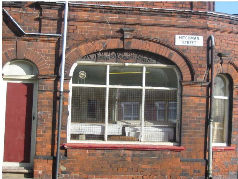
FIGURE 13: Shop window with decorative terracotta panels below arch.
