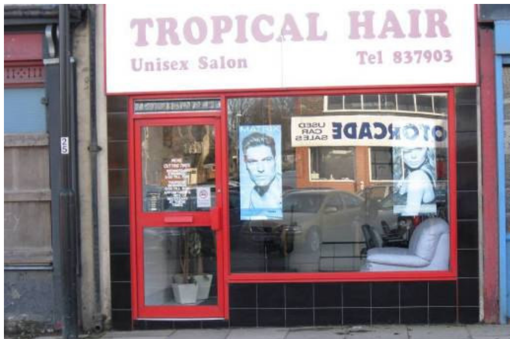
Examples of altered shopfronts where large signs or modern unsuitable shopfront and door including rollershutters.
