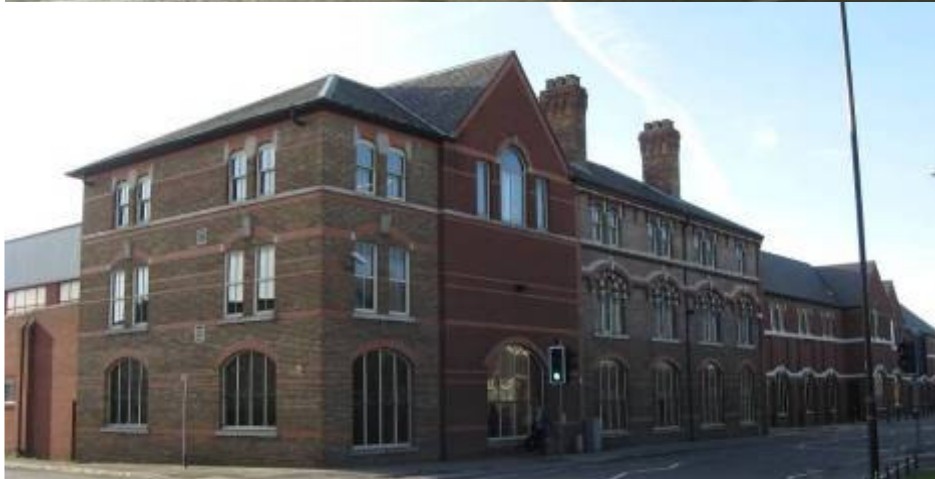
Before and after photographs showing what was removed in the 1990's to enable the extension of the Steelite factory.
