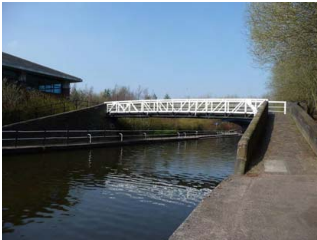
Fig. 31: View of Bridge 118 from southern approach
