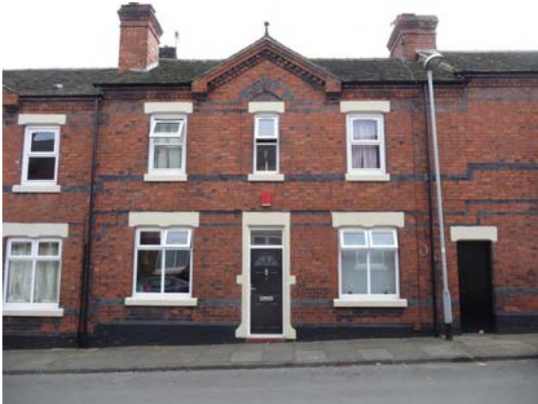
Fig. 17: Double fronted housing on Maddock Street housed managers and designers who worked at the Middleport Pottery
