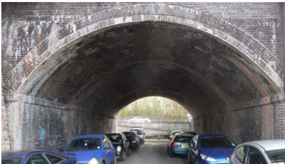
Fig. 46: Car parking underneath a railway arch
