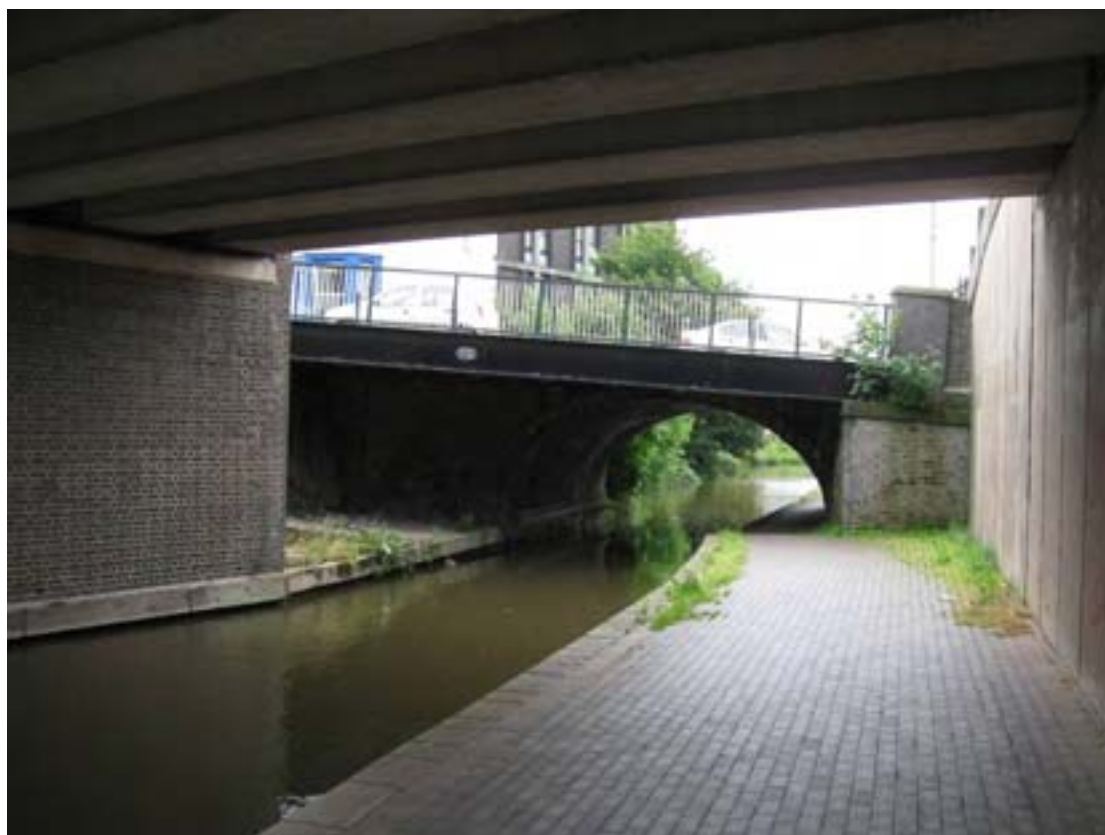
Fig. 48: The view of Glebe Bridge from the northern approach
