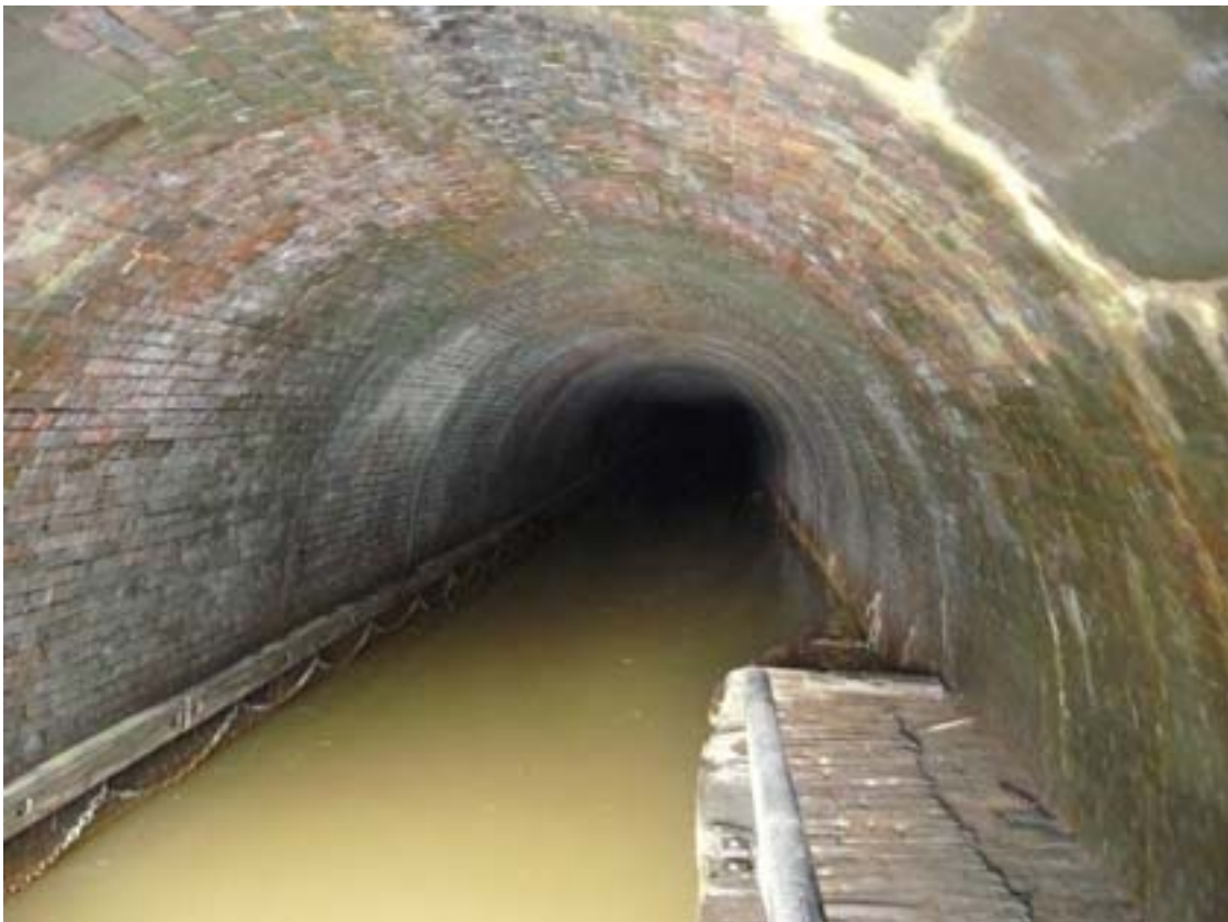
Fig. 1: Interior of the Harecastle Tunnels, as viewed from the southern entrance
