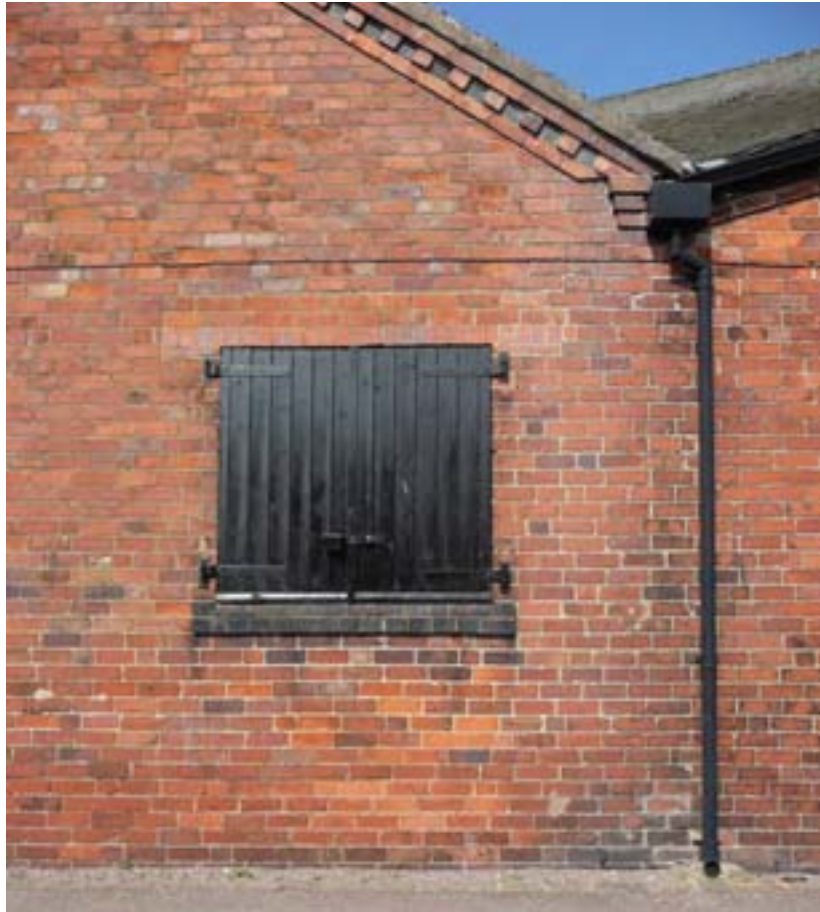
Fig. 37: Timber shutters to window with dentil finish to gable
