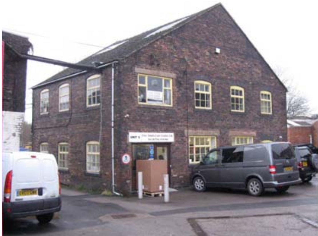
Fig. 11: Industrial building with painted window frames with segmental arches
