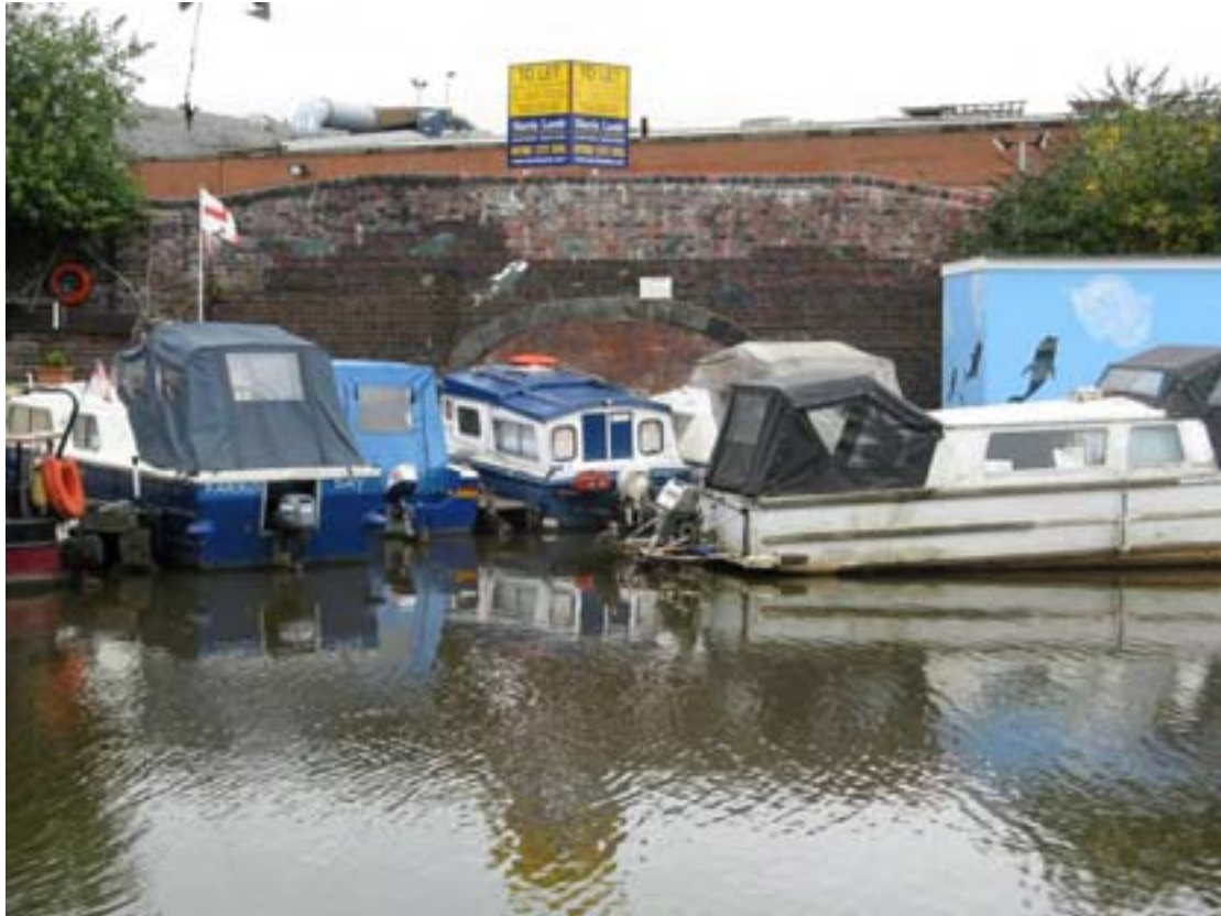
Fig. 49: Bricked up entrance to the former Stoke Basin
