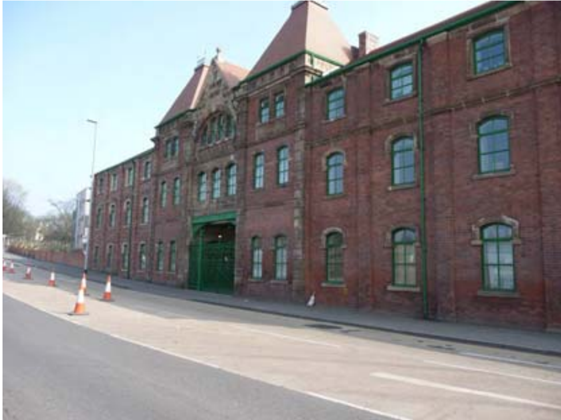
Fig. 35: Front elevation of former Cliffe Vale Pottery Works, as viewed from Shelton New Road
