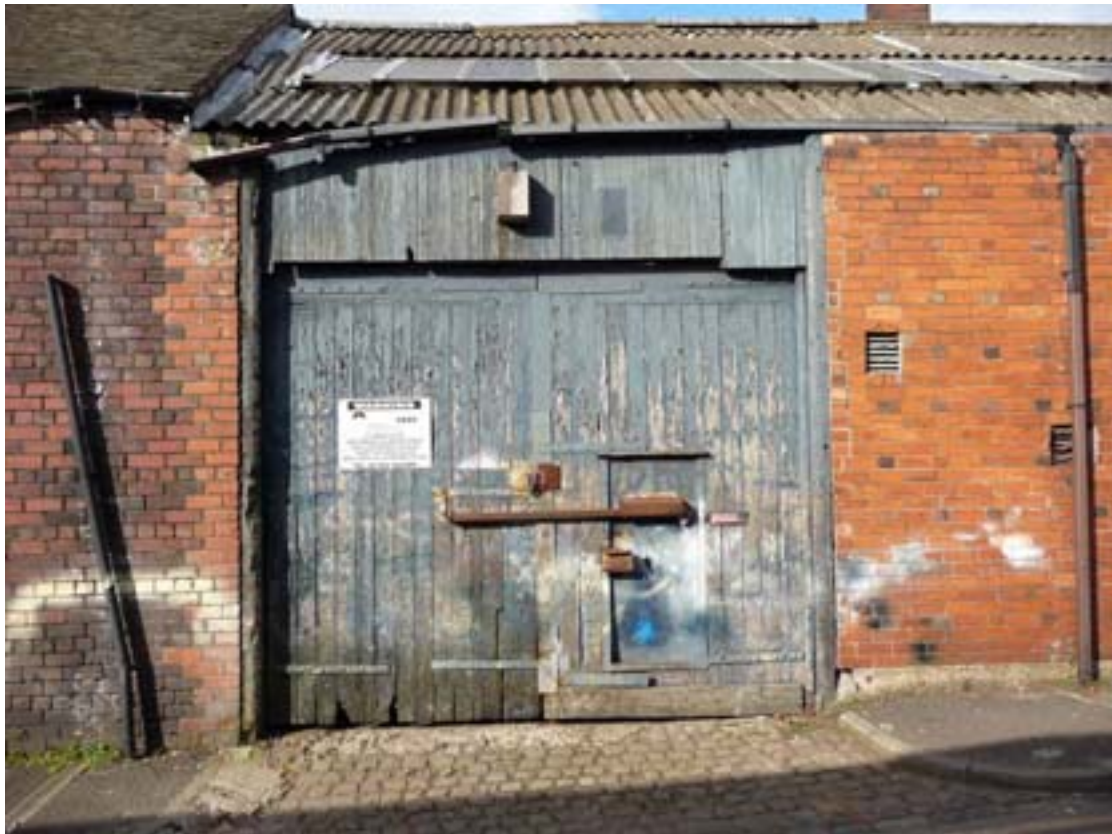
Fig. 24: Original timber doors mark a cart entrance from Longshaw Street
