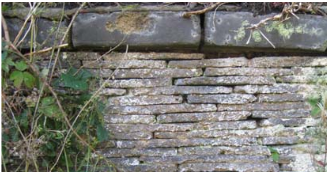
Fig. 25: Staffordshire blue Rosemary tiles and square copers constitute vernacular walling
