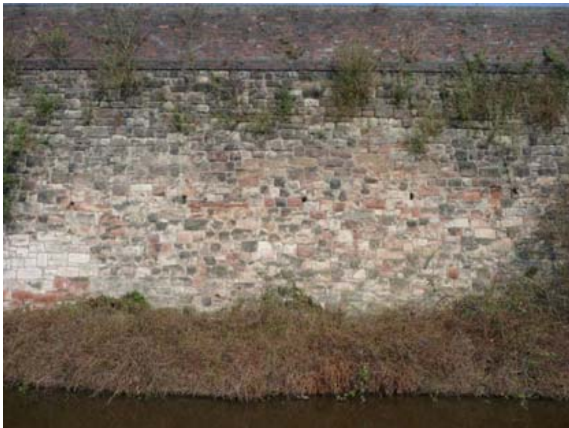
Fig. 43: Stone retaining wall to edge of canal
