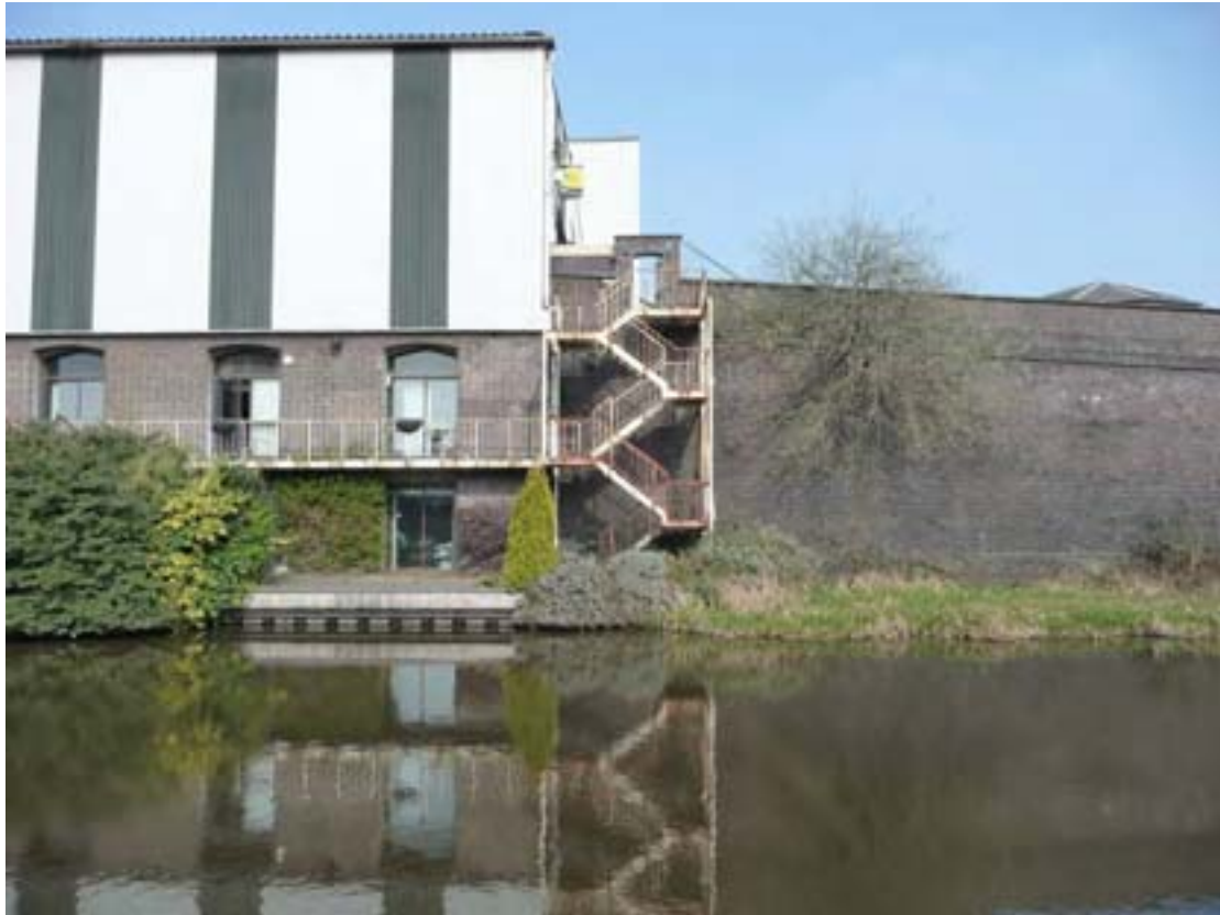
Fig. 41: Swift House, external metal fire escape and brick retaining wall
