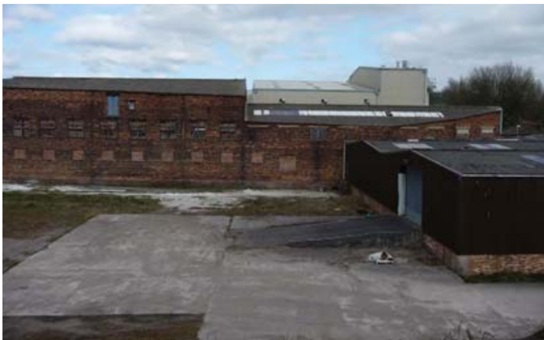
Fig. 14: Original warehouses still line the former Burslem Port Basin, now filled in
