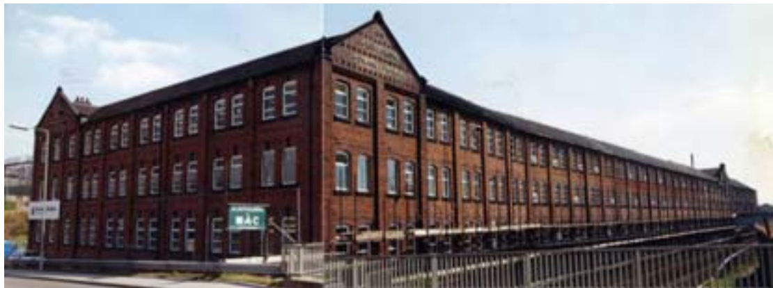
Fig. 51: Winkle & Wood's Colonial Pottery prior to demolition
