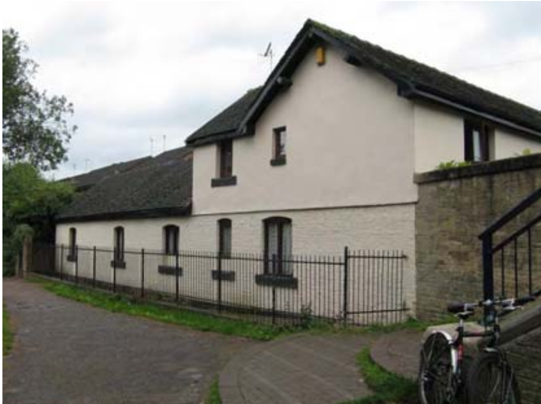
Fig. 58: Side elevation of Canalside Cottage adjacent to the canal
