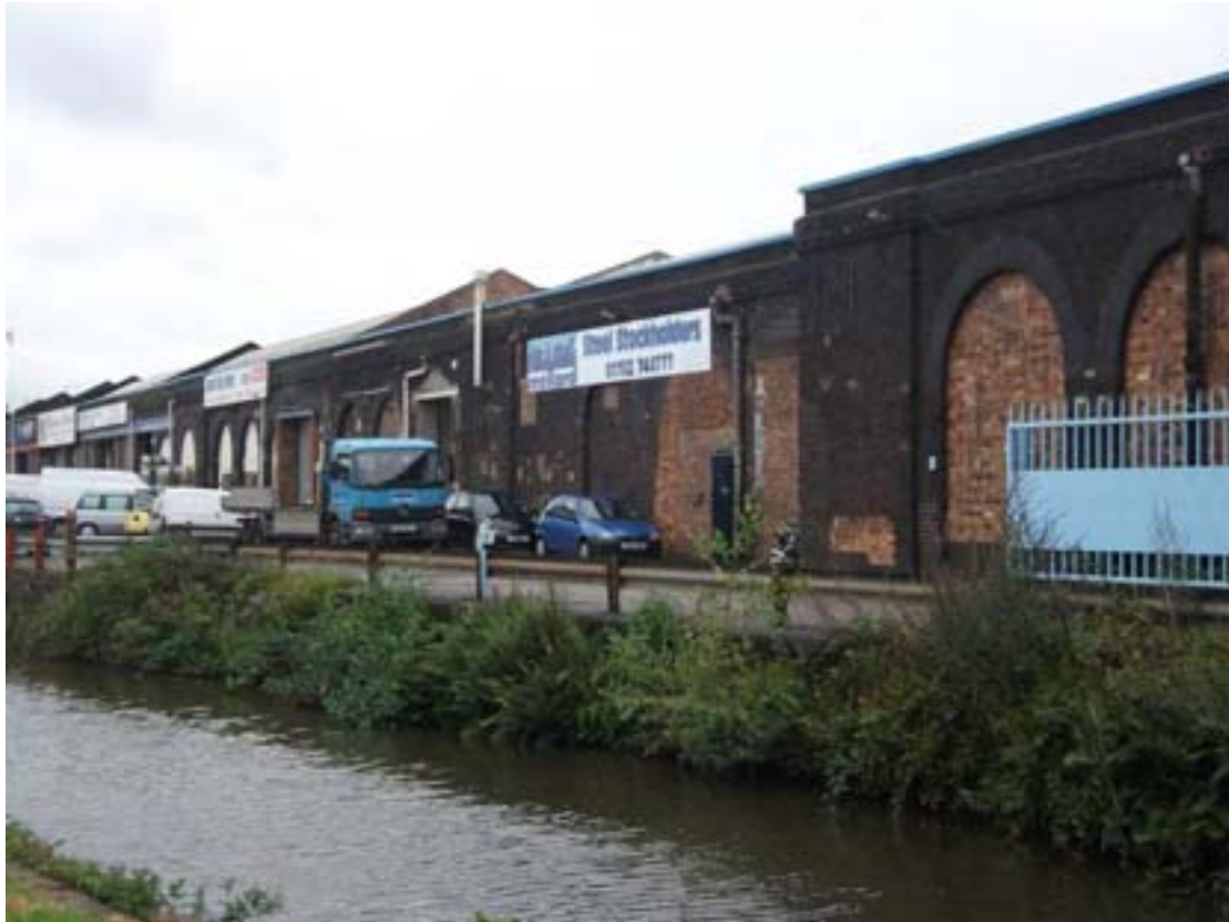
Fig. 50: The former railway shed adjacent to the canal
