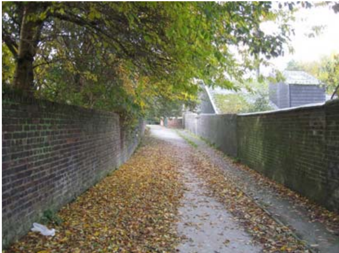
Fig. 39: The approach to the canal from Lower Bedford Street
