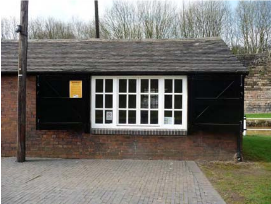
Fig. 4: Double casement windows to small building at Harecastle Tunnels, with Staffordshire blue clay paviours in the foreground
