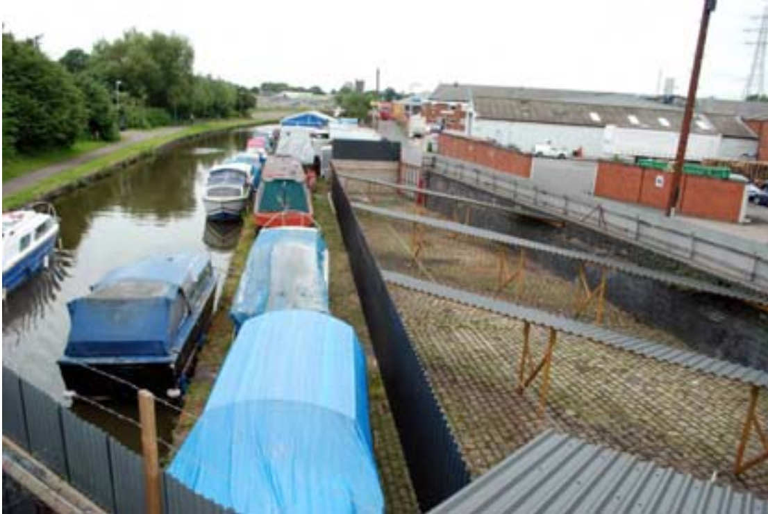
Fig. 53: Stone sett paving defines the former Stoke Basin Wharf
