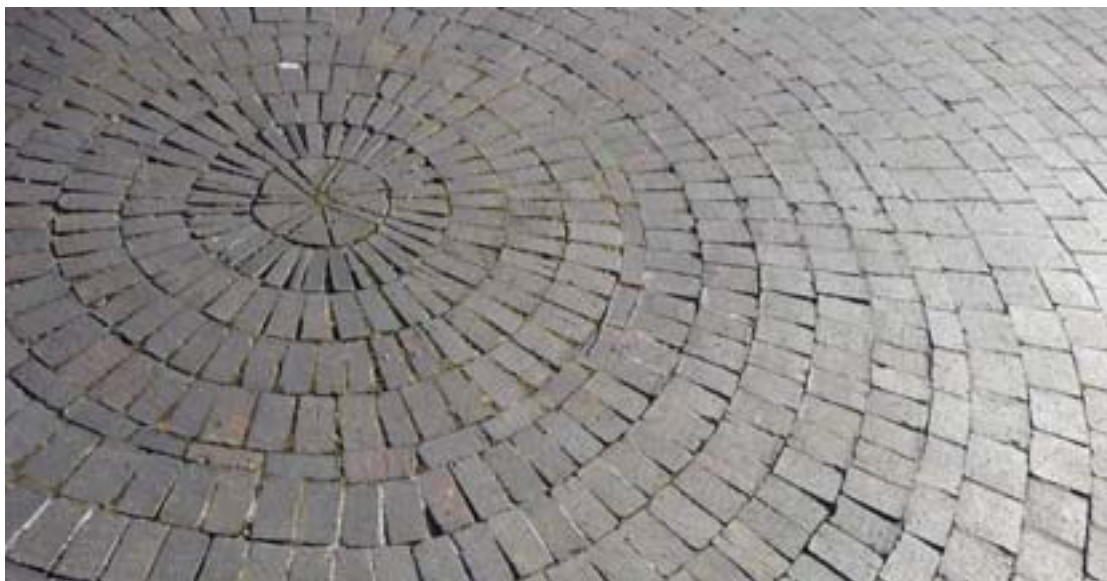
Fig. 55: Sett paving marks the junction of the towpath with the public footpath to Hanford
