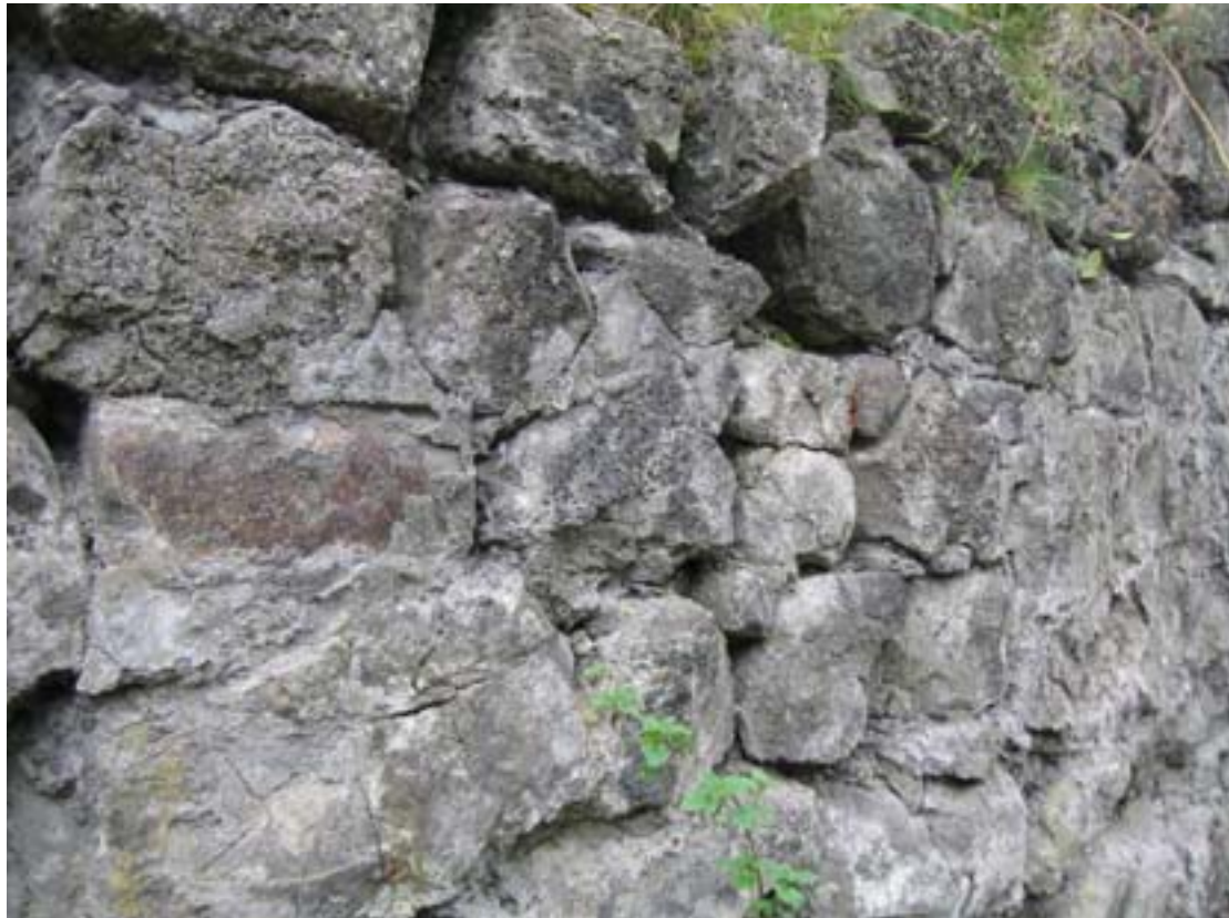
Fig. 6: Slag walling adjacent to the Ravensdale Playing Pitch
