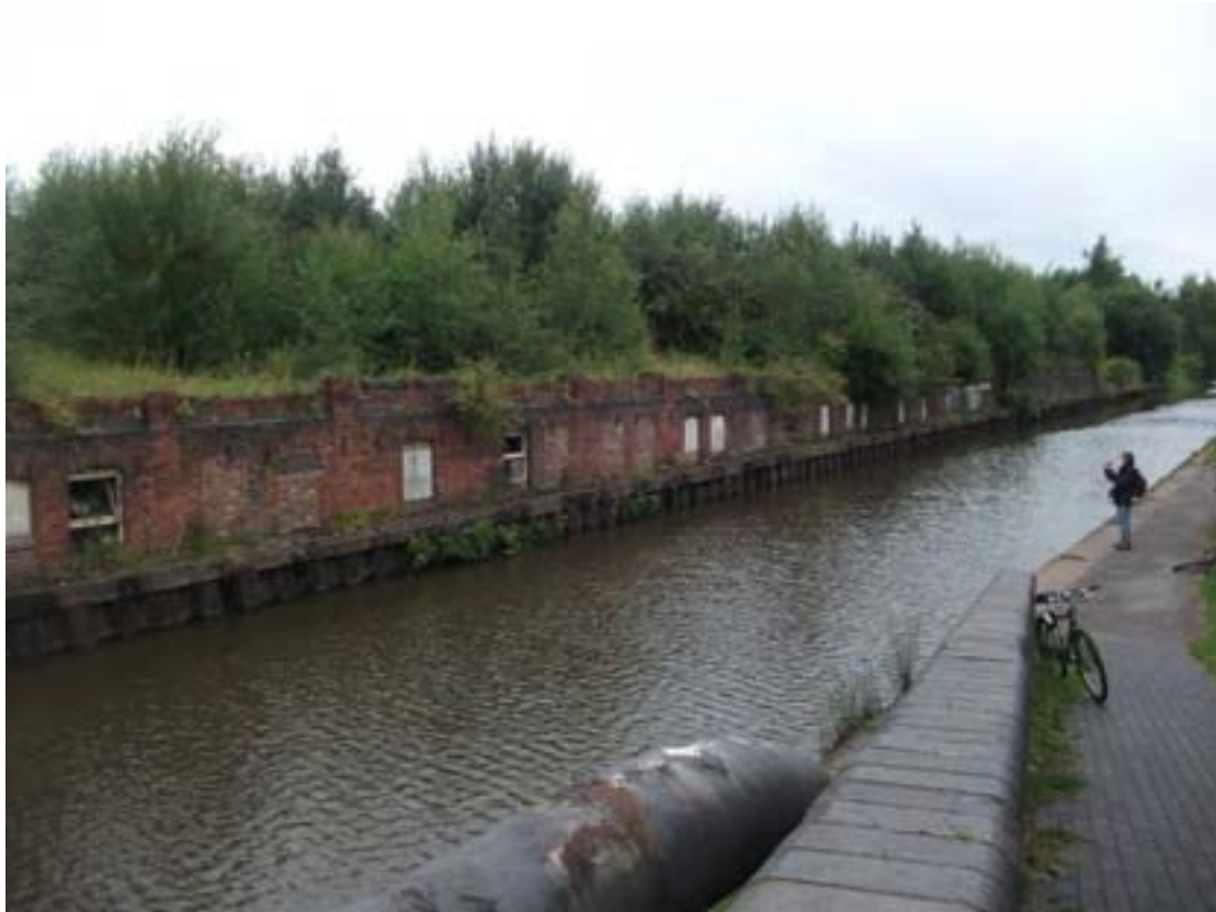
Fig. 52: The remaining elevational fragments of the former Colonial Pottery
