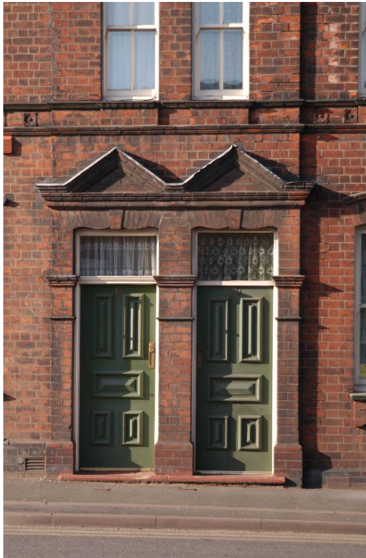
FIGURE 14: Doors with the simplest brick door-case.
