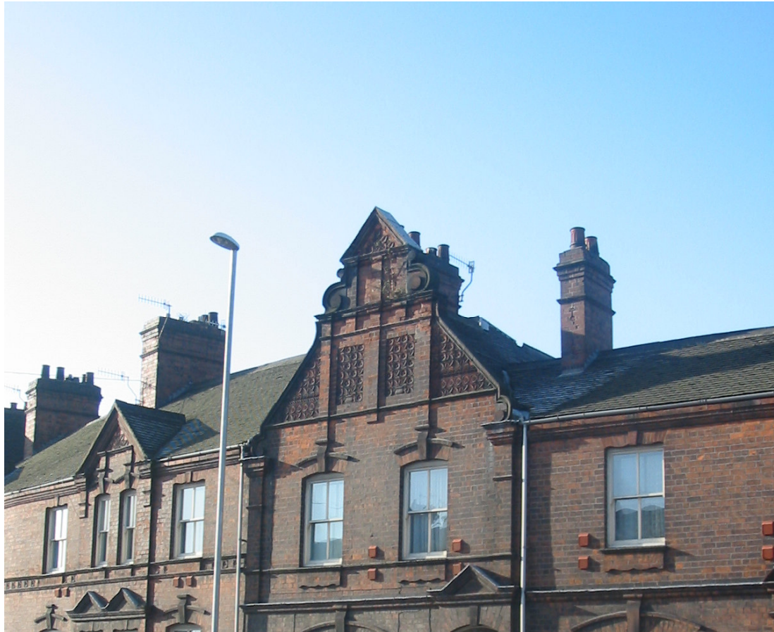
FIGURE 12: Roofs, chimneys and original moulded chimney pots
