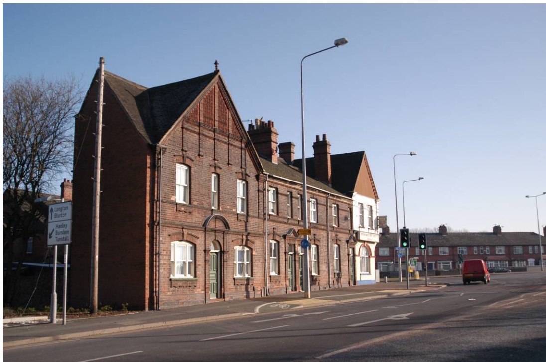
FIGURE 9: View from City Road
