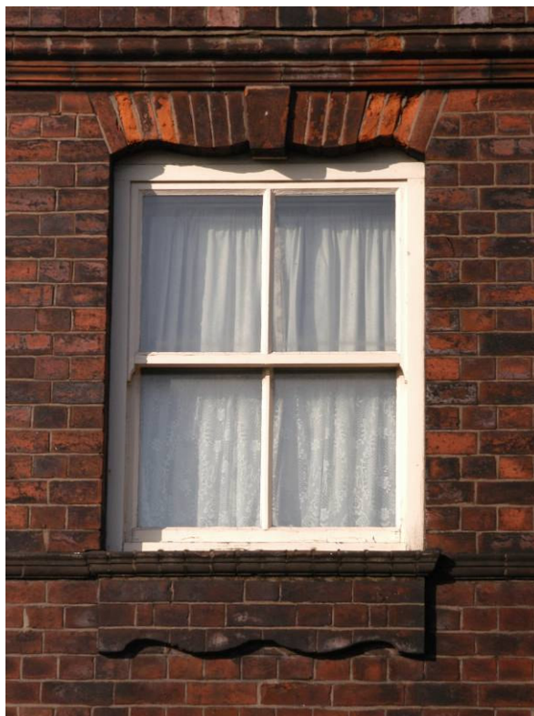
Figure 13: Windows with moulded aprons and curved arches
