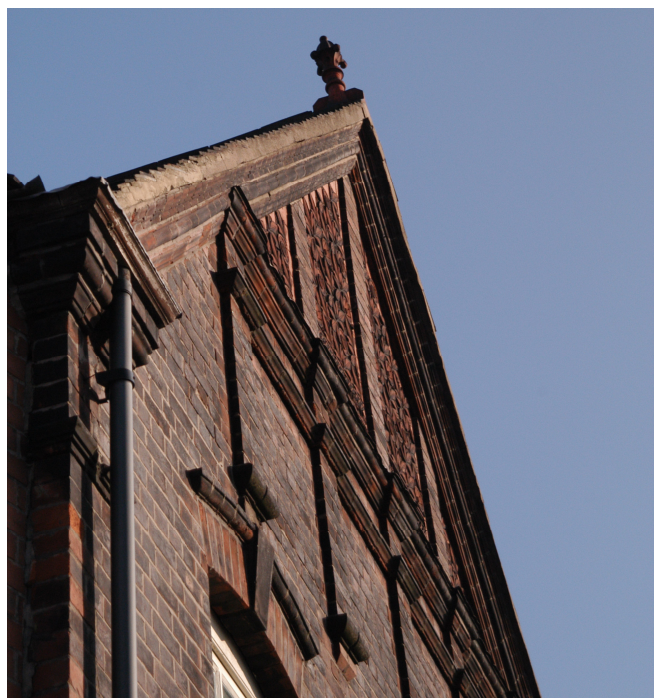
FIGURE 11: Moulded brickwork used to great effect in gable
