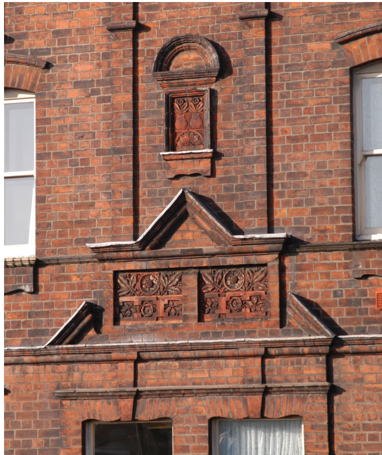
FIGURE 15: Detail from larger door-case showing decorative brickwork over door fanlights
